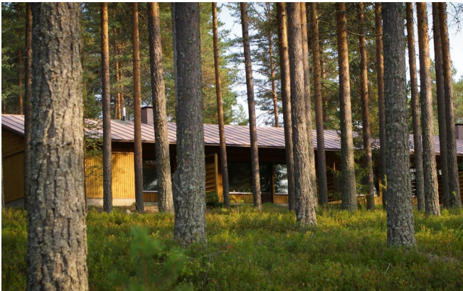
The row house among the pines
