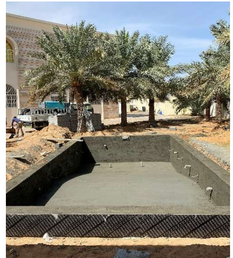
Pool shell preparation
