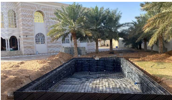
Reinforcement and pool shell works
