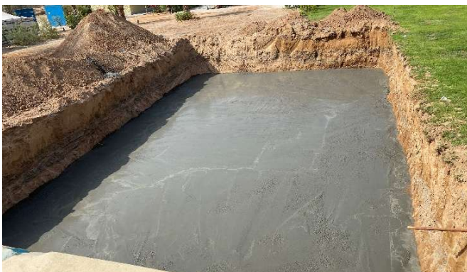
Concrete base preparation
