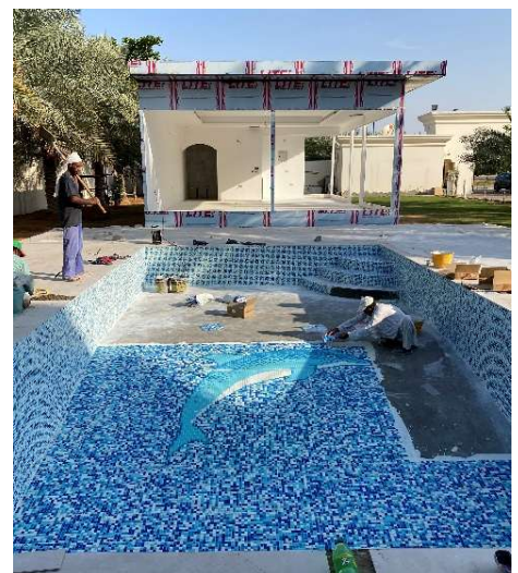
Mosaic installation in progress
