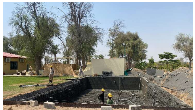
Reinforcement and embedded pool pipework
