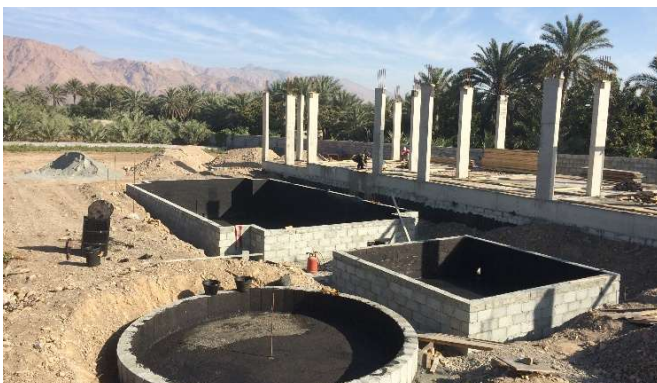
Pool and spa structures during construction
