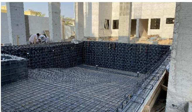
Waterproofing and reinforcement stage
