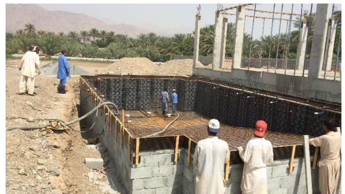
Formwork and reinforcement stage
