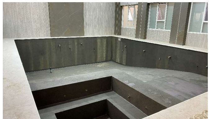
Pool shell and internal steps before finishing
