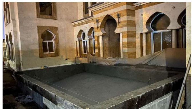
Pool body before mosaic and cladding finishes
