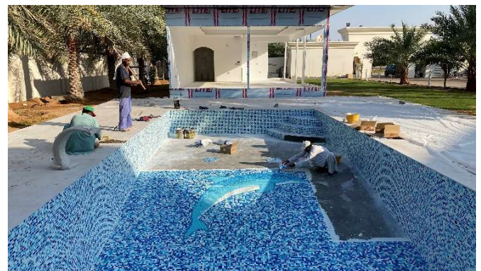
Mosaic finishing in progress
