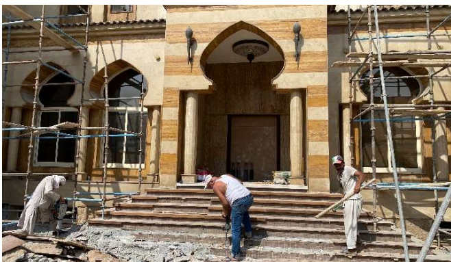
Site preparation and excavation
